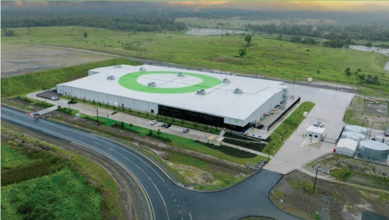
In April, Fortescue officially opened an electrolyzer manufacturing facility in Australia – one of the first globally to house an automated assembly line.
